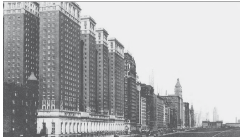
An inhabited wall faces the empty field of the railway yard. Michigan Avenue, Chicago
